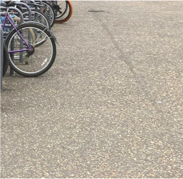
Vehicular grade asphalt with rolled buff chippings
