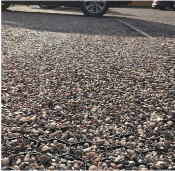
Permeable gravel retention surface
