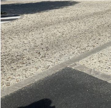
Insitu exposed aggregate concrete with sett band
